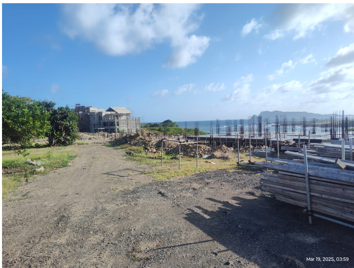
Figure 2: User-supplied ground-level image bearing an in-frame timestamp of 19 March 2025. It shows unfinished concrete works, exposed reinforcement, formwork/materials and no visible workers in that single frame.
